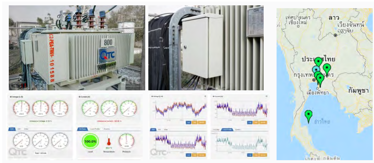
QTC Smart Transformer Function Model
