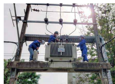
Smart Monitoring Box Set Installation in the Trial-Use Agreement
