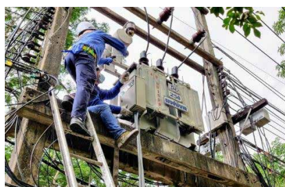
Smart Monitoring Box Set Installation in the Trial-Use Agreement
